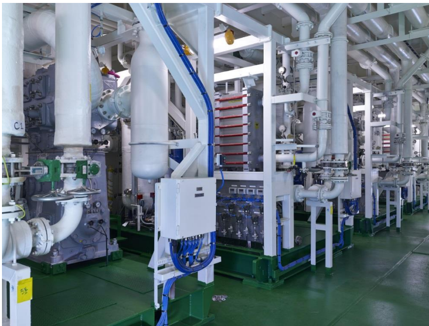
Figure 3: Laby ® Compressor system installed on an LPG carrier
